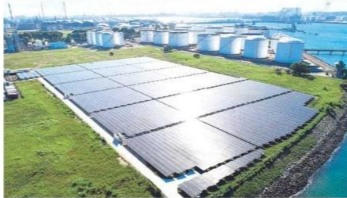
JTC Corporation currently has solar panels on temporarily vacant land on Jurong Island (above), and on the roofs of more than 20 buildings, amounting to over 10MWp of installed solar capacity. It expects to increase this capacity to 100MWp within the next three years by using more rooftops and vacant land for solar deployment.
