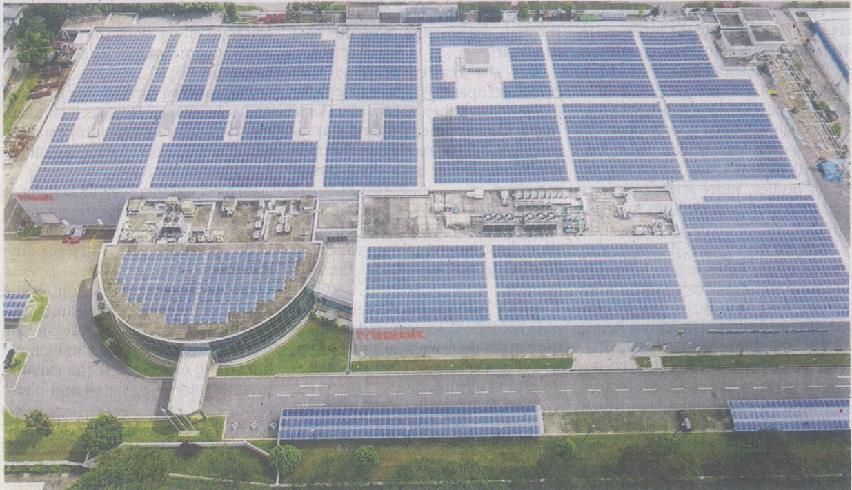
Yamazaki Mazak Singapore has partnered Cleantech Solar to operate a 16,000 sq m system of 6,000 solar panels on the rooftop of its facilities to power up to 35 per cent of the new manufacturing plant's power needs.
